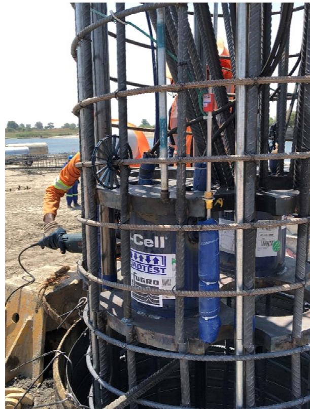
Assembly being lowered into the pile bore
