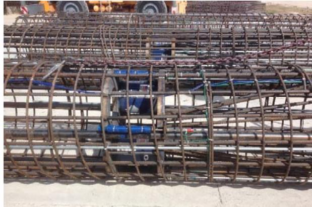
O-cell cage ready for installation into the pile bore
