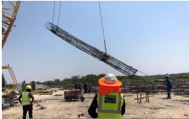
O-cell cage lifting into place ready for installation into the pile bore
